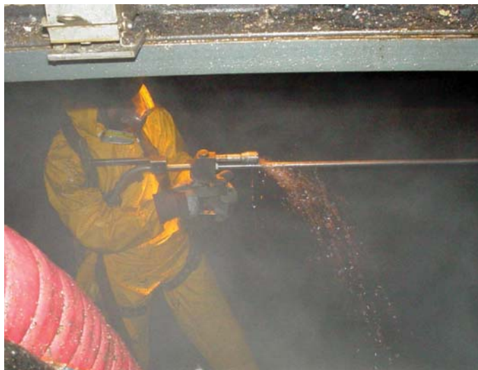
A MPW technician uses waterblasting technology in a confined space to remove debris from a customer site. MPW entered the waterblasting business in 1972, by cleaning kettles and reactors in paint and resin manufacturing industries.
